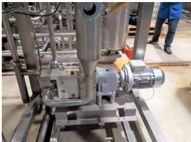
Pumped liquid - SLES 70%; 3 bar; 6 m 3 /h Pump - LPX50-2
